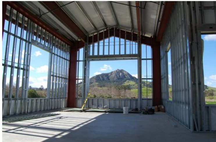
Interior Space of Technology Park Lab 2B - Construction Photo February 2010
